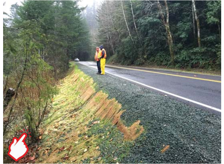
FIGURE 8b Agness Road site after deep-patch construction in December 2014.
