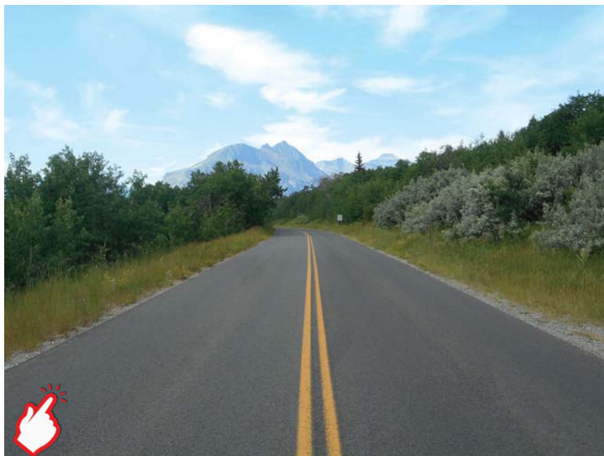
FIGURE 3b After photograph in July 2017 showing GTSR deep-patch location
