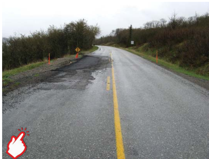
FIGURE 3a Before photograph in May 2011 showing GTSR deep-patch location.
