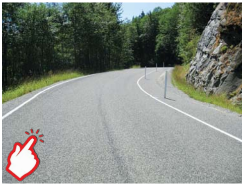
FIGURE 5b After photograph in July 2017 of the MFSRR Milepost 10 deep patch.
