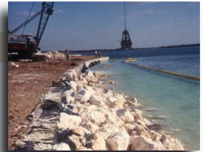
Monofilament with Riprap
