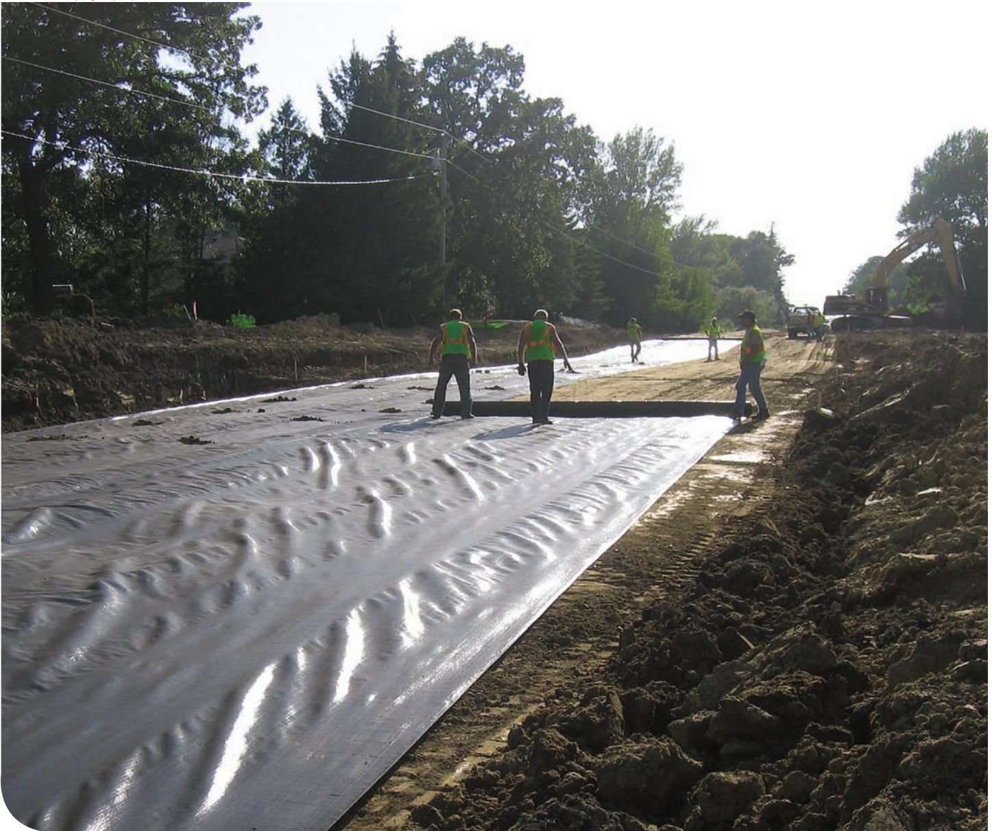
Photos | Geotextile being rolled out to provide separation.
